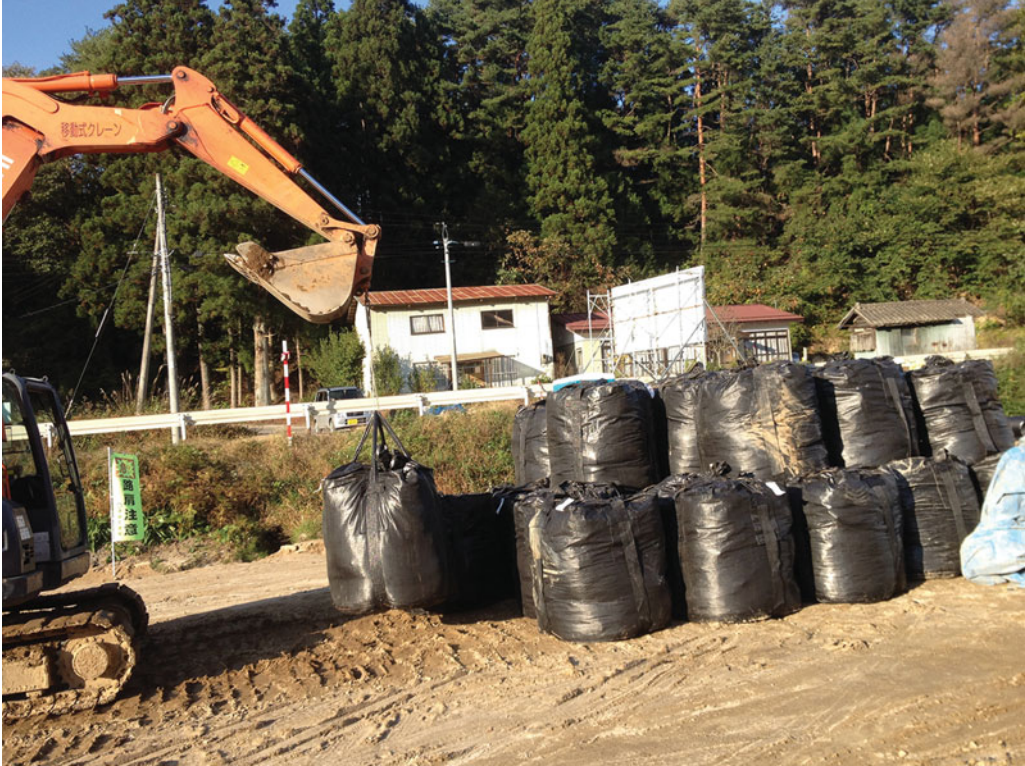
Figure 6. A small-scale temporary storage site for contaminated soil, near Minamisōma (photograph: Jean-Paul Demoule, October 2013).
