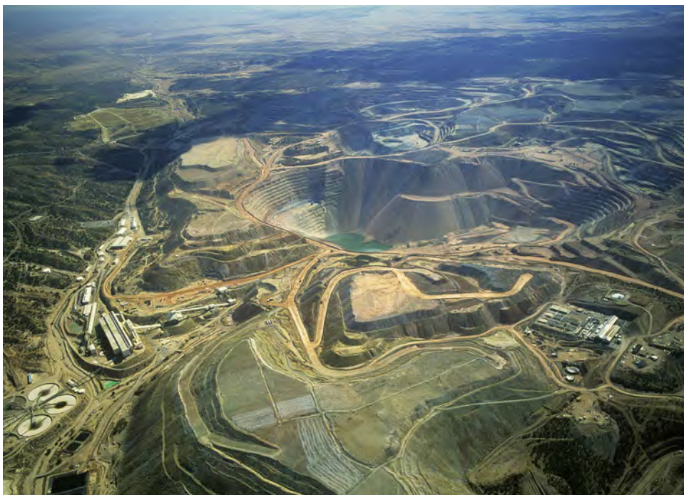
Fig 4: Tyrone open-pit copper mine, photographed in 2001. Many of the mesa-like forms surrounding the pit have since been reshaped and reclaimed since the making of this image. Image courtesy of aerial photographer Jim Wark
