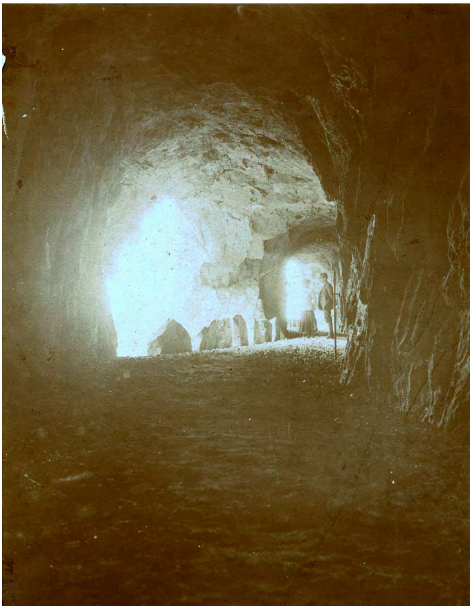
Tunnel work by the Jøssing fjord. Image from Road Director Hans H. Krag's photo album, 1900. Image courtesy of the Norwegian Road Museum.
