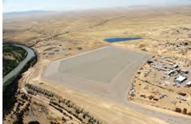
Shiprock Disposal Cell, NM.
