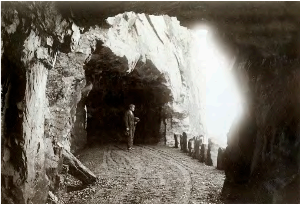
Road construction Saude-Storhjet. Image from Road Director Hans H. Krag's photo album, 1900. Image courtesy of the Norwegian Road Museum.
