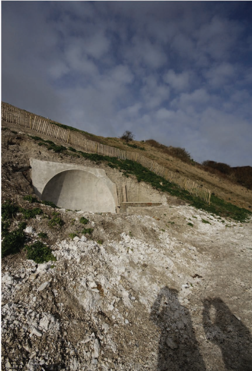
FIGURE 10 Recently uncovered sound mirror at Fan Bay, Kent. The mirror was carved into the chalk cliff and then lined with concrete.
