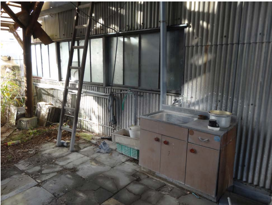
FIGURE 2. A sink with a washed mug, which was in the same position when I revisited the site in September 2016.
