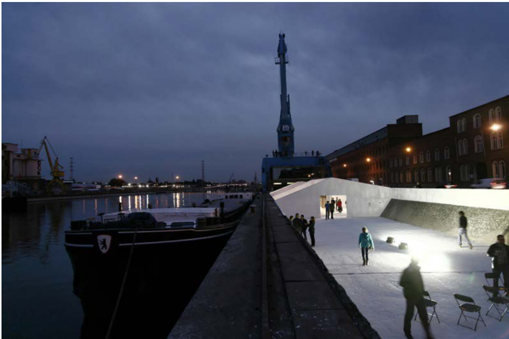
FIGURE 1. The site of the Grindbakken exhibition: a reconverted series of former gravel containers in the old harbour of Ghent (photograph by Rotor).
